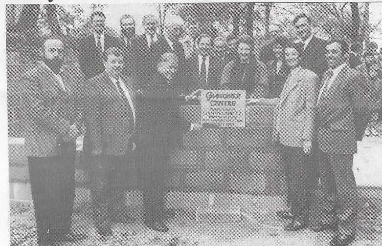
At the laying of the foundation stone for the new Granuaile Interpretative Centre in Louisburgh, front L - R Cllr. Frank Chambers, Mr John Kilcoyne, Minister Mr Liam Hyland, Author Anne Chambers, Mr John Burke (Building Contractor), Back Mr Tony Cawley, FAs, Mr Paul Kirkpatrick, Chief Exec. South west Mayo Leader Group, Mr Michael Moran, Chairman SWMLG, Mr sean Harney, Louisburgh Development Company, Mr Dermot Power Dept of Agriculture, Cllr Michael Ring, Mr Tonny Joe Duffy, Fr Paddy Mooney, Mrs Clementine Lyons, Chariperson, Louisburgh Development Company, Mr Vincent O'Loughlin and Deputy Seamus Hughes
